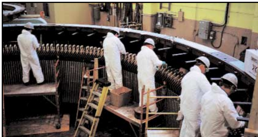
Turbine repair at Brilliant Dam.
