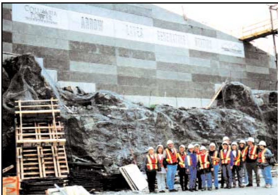
Columbia Basin Trust staff tour the construction site of the new Arrow Lakes Generating Station.
