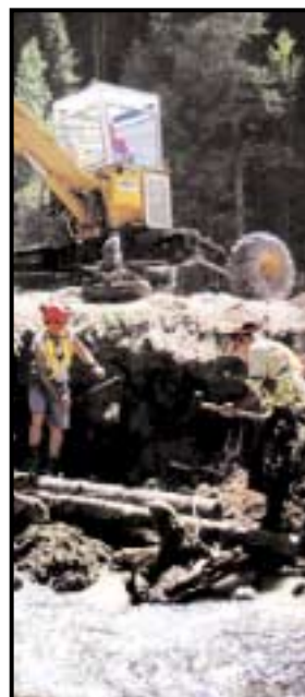
WINDERMERE: Spyder Hoe and hand labour crew complete installation of rootwads along Windermere Creek.
