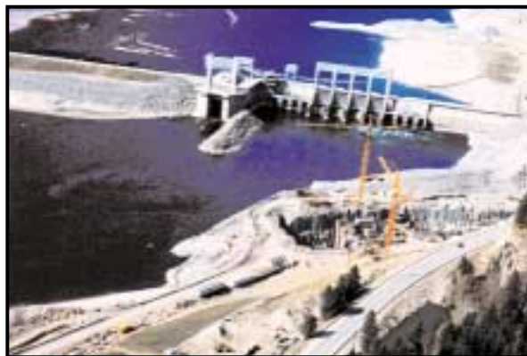
Arrow Lakes Generating Station at Keenleyside Dam.
