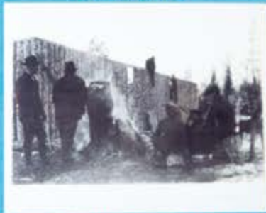
erecting old Grasmere Hall
