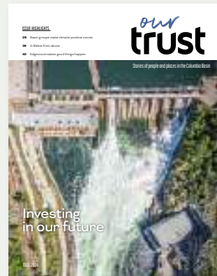
Cover Photo: Brilliant Dam and Brilliant Expansion Generating Stations on the Kootenay River by Adrian Wagner.
