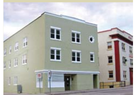
CBT helped support mechanical upgrades at Sanctuary House in Trail.
