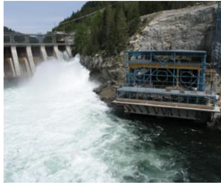
Brilliant Dam and Brilliant Expansion Project
